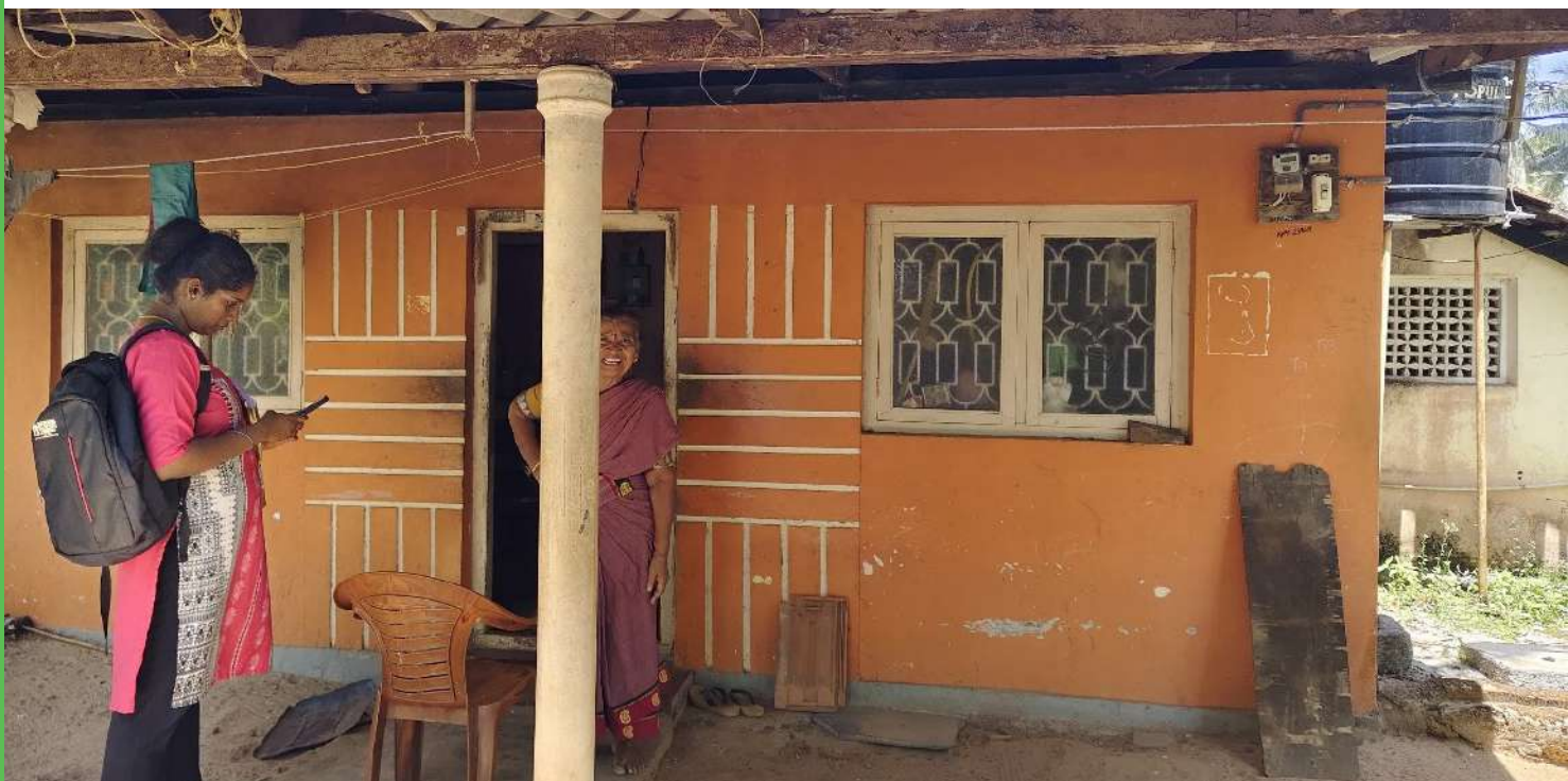
A semi-pucca house with an asbestos sheet roof, Data Collection at Udupi, Karnataka.
